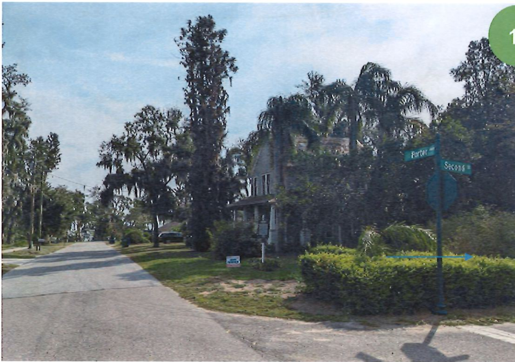
Looking down Porter Ave from Second St. near the historic Harper home on the National Register of Historic Homes; substandard roadway lacking proper pavement thickness, curbs and gutters, no sidewalk; no trail connection. F.S. 163.340 Factors evidenced: (a), (d).
