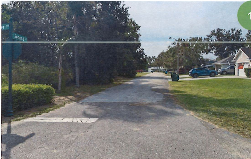
Looking down Second St from Porter Ave; substandard roadway lacking proper pavement thickness, curbs and gutters, no sidewalk; no trail connection. F.S. 163.340 Factors evidenced: (a), (d).
